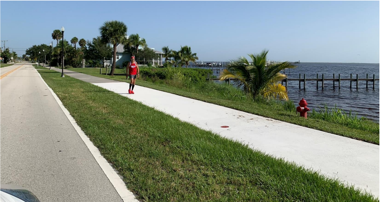
Figure 7 - A view of the sidewalk along Indian River Drive
