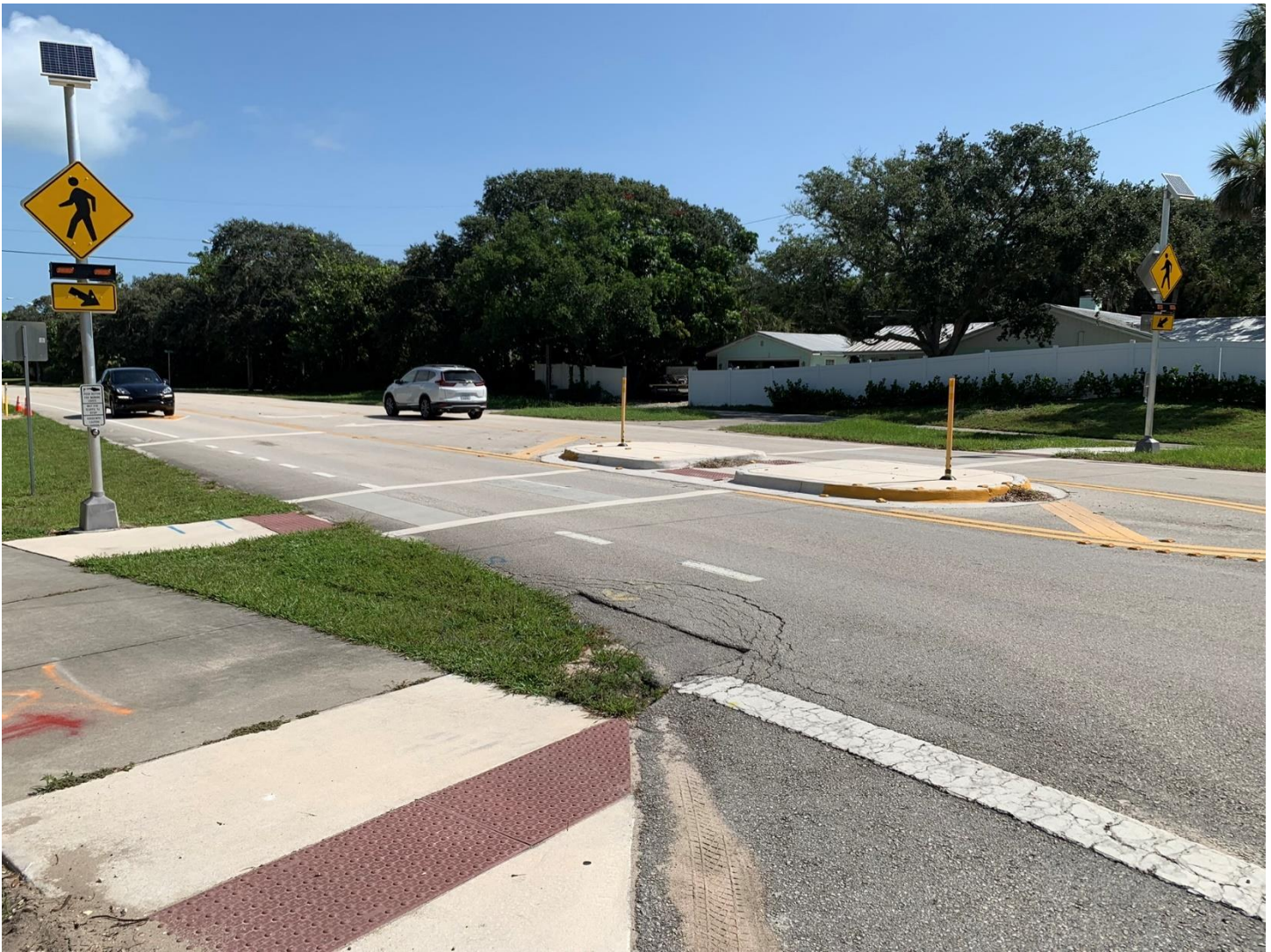
Figure 6 - Crossing Location on SR A1A
