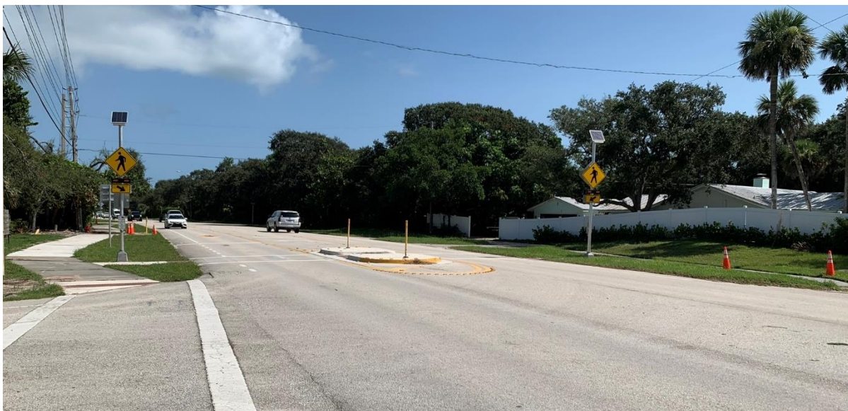
Figure 10 - A pedestrian crossing on SR A1A near Greytwig Road
