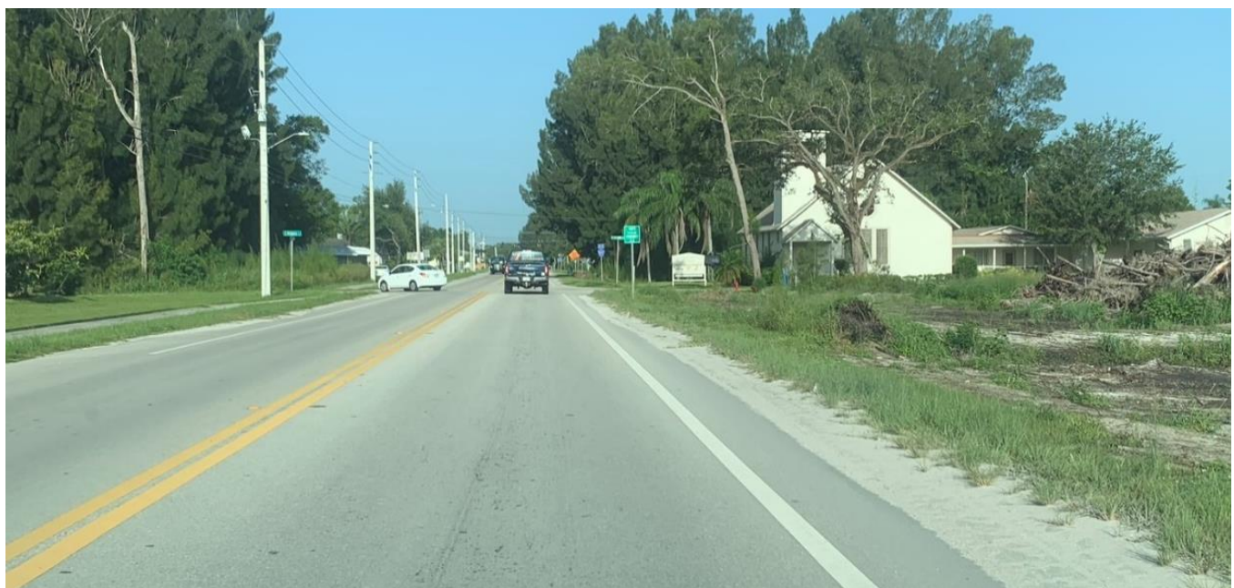
Figure 12 – Sand and grass encroaching on bike lane, westbound on CR 512, near N Hickory Street in Fellsmere
