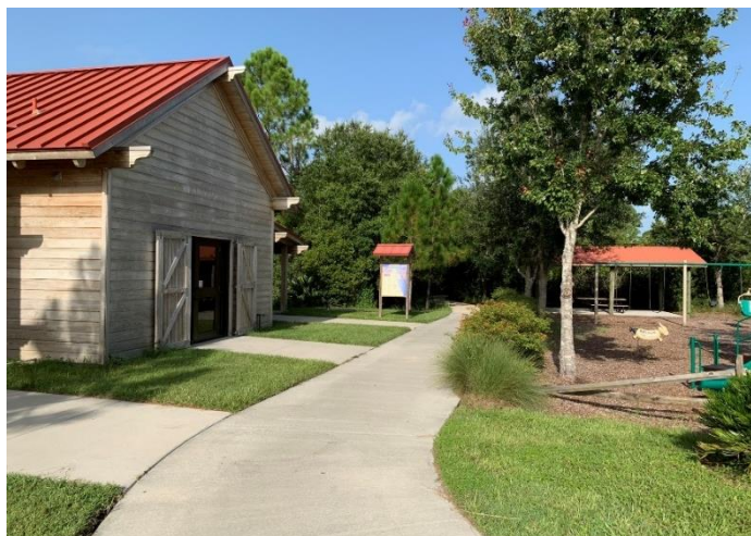
Figure 13 – Fellsmere Trailhead Preserve Information Center and playground
